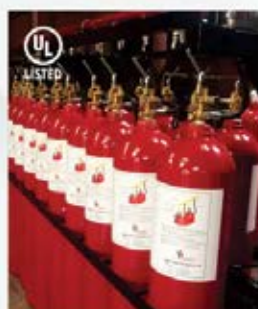
CO2 Fire Extinguishing System
