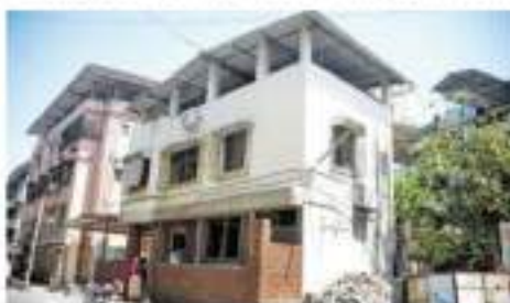
Work going on in the ground floor of the Vasai-Virar City civic commissioner's bungalow. PHOTO: MITTEL
